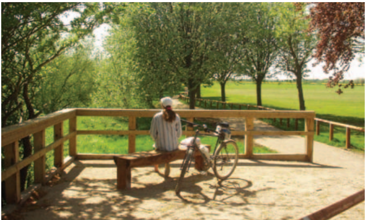
Figure 22: The path after completion of the scheme.
