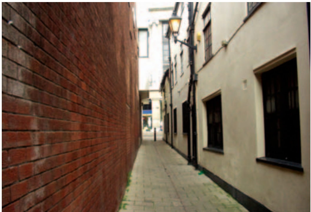
Figure 1: Historic alleyway within the City centre, near to the Old Market Square. This alleyway runs between St Peters Gate and the Poultry and dates back to c 1850's.
