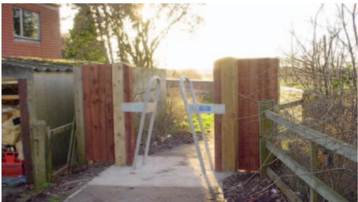
Figure 25: Motorcycle Inhibitor Barrier on a “shared use” pedestrian and cycle path in an urban setting.
